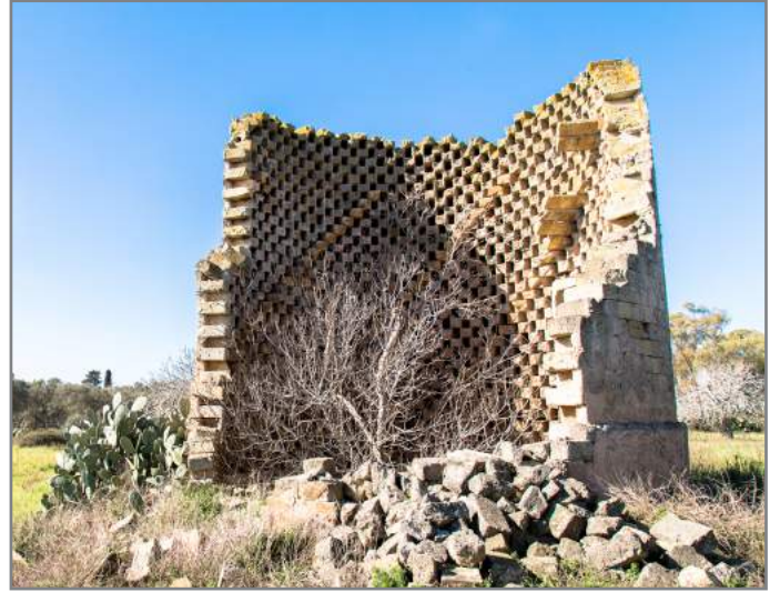
Torre colombaia Dovecote tower
