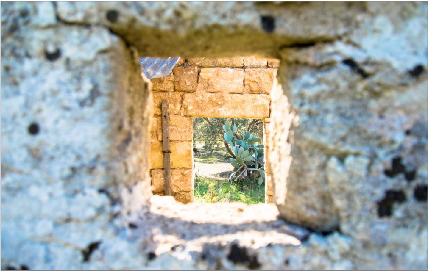
Torre colombaia Dovecote tower
