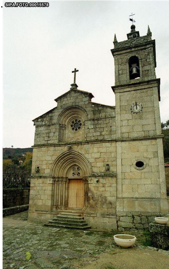
Figure 4 – Barrô parish church, Resende. 17
