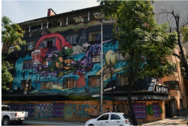
Figure 5. The façade of Chanti Ollin following the eviction, 2017
